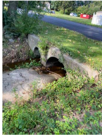
Brookside/Glenbrook Culverts Downstream
