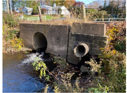
Derby Milford Culvert Downstream
