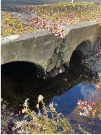
Brookside/Glenbrook Culverts Upstream
