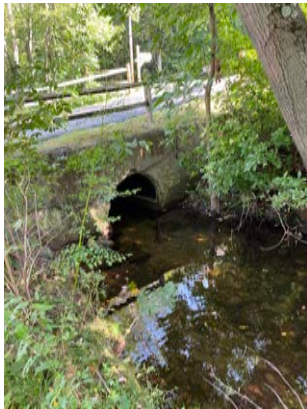
East Slope Driveway Culvert-Downstream
