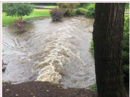
Downstream of Railroad culvert
