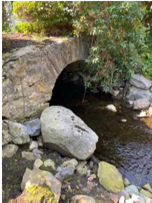
Derby Milford Road Culvert Upstream
