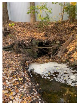
Railroad stone culvert-Upstream
