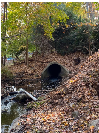
Looking at 48" culvert discharge upstream of railroad culvert
