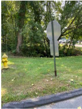
Peck Lane looking at culverts discharge pt
