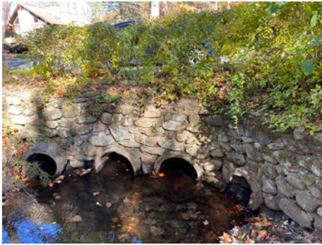
Coachmans culverts discharge
