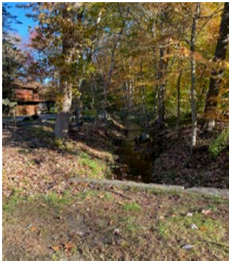
Coachmans culverts-looking upstream
